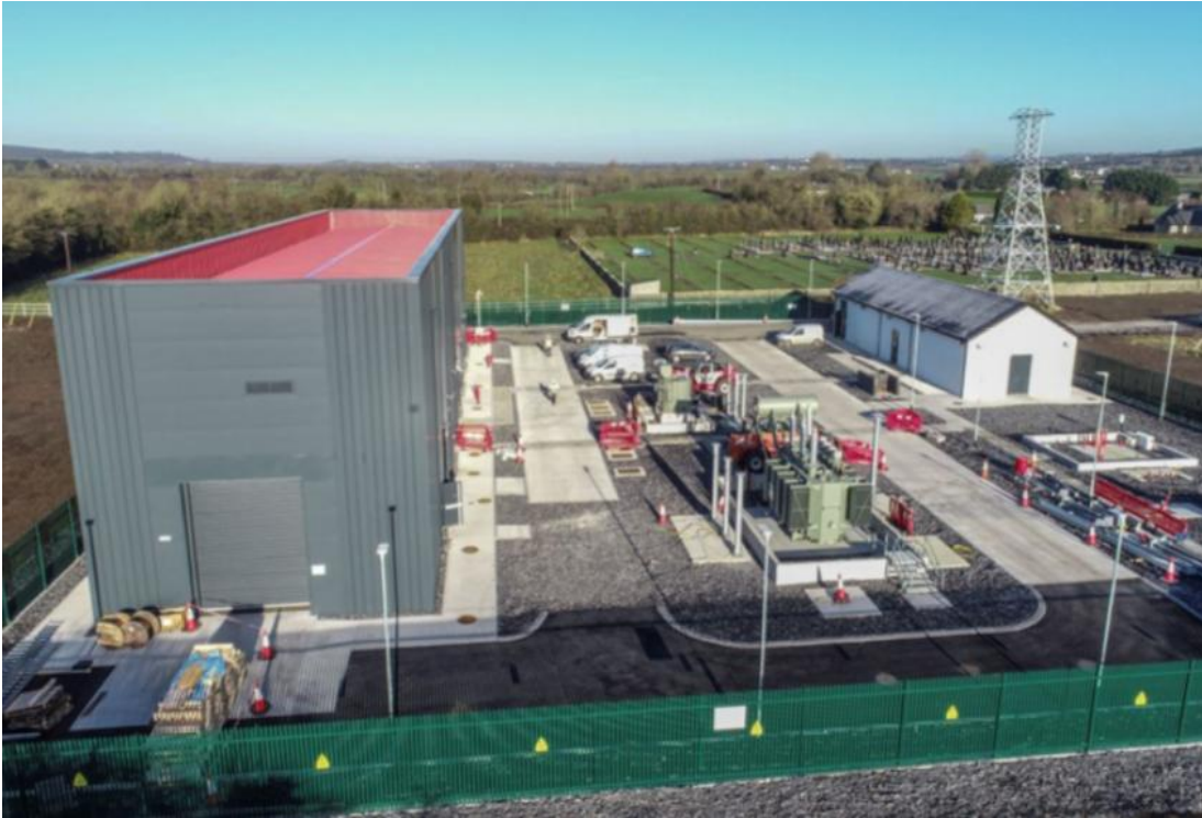
Typical 110 kV GIS Substation
